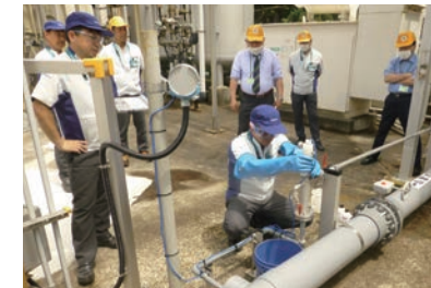
Risk assessments by on-site verification
