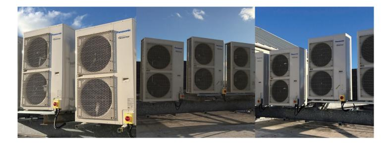
units were installed outdoors, whilst four under-ceiling units and four wall-ducted systems were established indoors. A further 28kW of PACi cooling technology have been specified to be installed within the factory.
