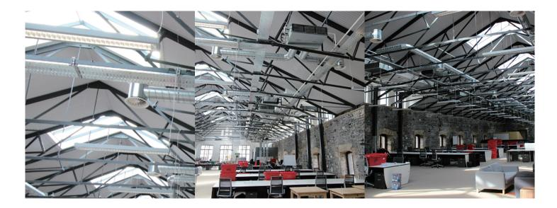
During the summer months the system allows for a purge during the night, allowing the cooler night air to be present for a fresh start to the day. Adding to the efficiency of the system, the number of ERVs running at any one time can be reduced depending on the number of people occupying the space, for example, during lunch times.
