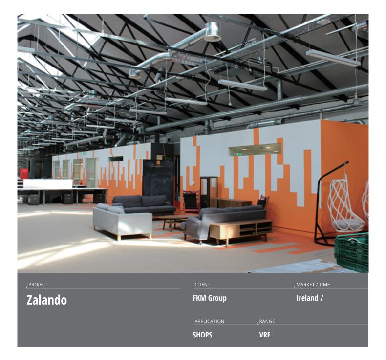
When online fashion brand Zalando required a sustainable, energy-efficient cooling solution for its 19th century warehouse office conversion at Grand Canal Quay, Dublin, FKM Group selected the Panasonic 3-pipe ECOi MF2 AC solution to be installed by Crystal Air. The project needed to be completed with minimal changes to the fabric of the building, with fresh air delivered using ERVs located in the roof space of the building.
