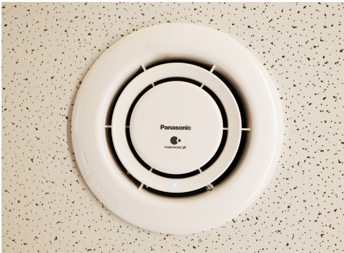
Neat installation of air-e ceiling mounted nanoe™ X generator.
