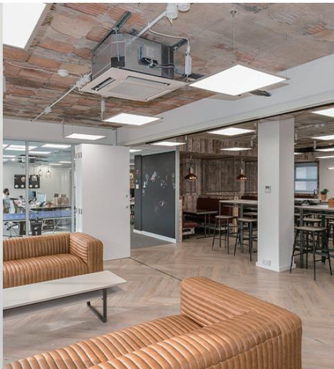
processes. For the end user, the benefit is that each cassette can be controlled individually, allowing one to be in cooling mode while the other is in heating mode.
