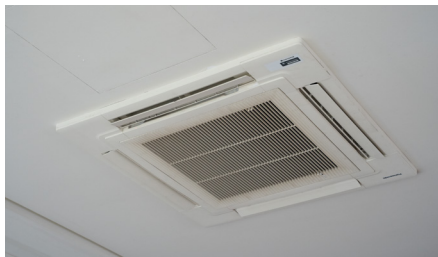
4-way cassette air conditioner equipped with nanoe™ X.
