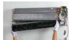
Removal of cross flow fan without lifting the evaporator
