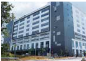
Malaysia Gaprana project
