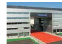
PAPARS Panasonic Appliances Air Conditioning & Refrigeration System (Gunma, Japan)
