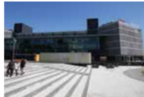
Spain PTA Malaga
