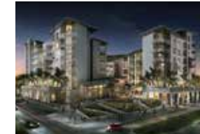
Panama Mosaic Building PANAMA PACIFICO
