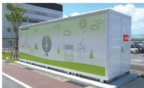
Storage battery container (Tokushima Factory)
