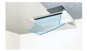
(1) One-direction "down-blow" system
