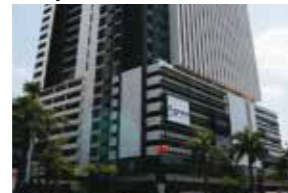
Malaysia Plaza 33 Office Block A
