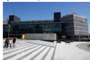
Spain PTA Malaga
