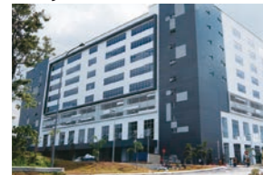
Malaysia Gaprana project
