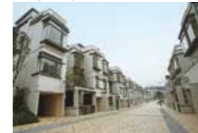
Hong Kong The Green Project
