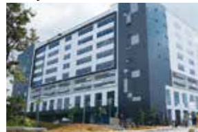
Malaysia Gapruna project
