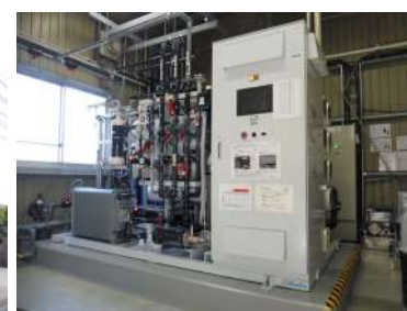
Water purification system with electrical resin regenerator
